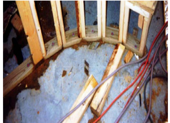
Fastening Wood Sill Plate to Concrete Floor
