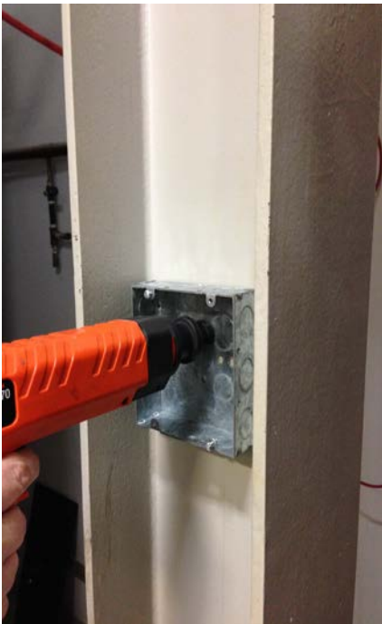
Electrical Box to Steel Beam
