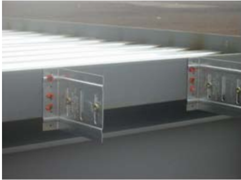
Light Gage Steel Fastened to Steel
